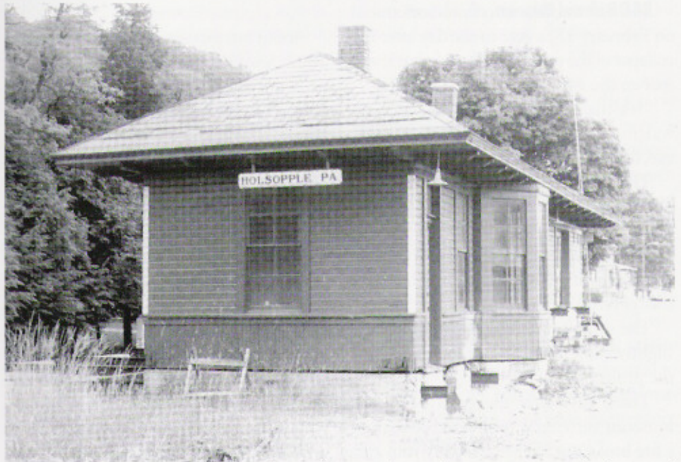
Hollsopple's second station, built after the first one burned in 1915, was jacked up and moved back from the tracks in 1980.
